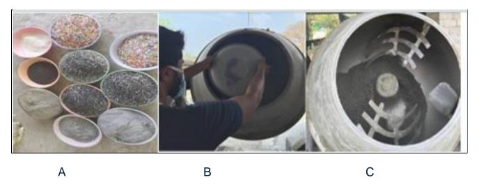
Fig. 2 showing making of final brick; (a) Batching of materials (b) placing of materials to mix machine (c) Mixing
