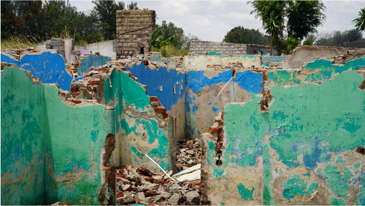
The demolition site by Lake Hawassa
